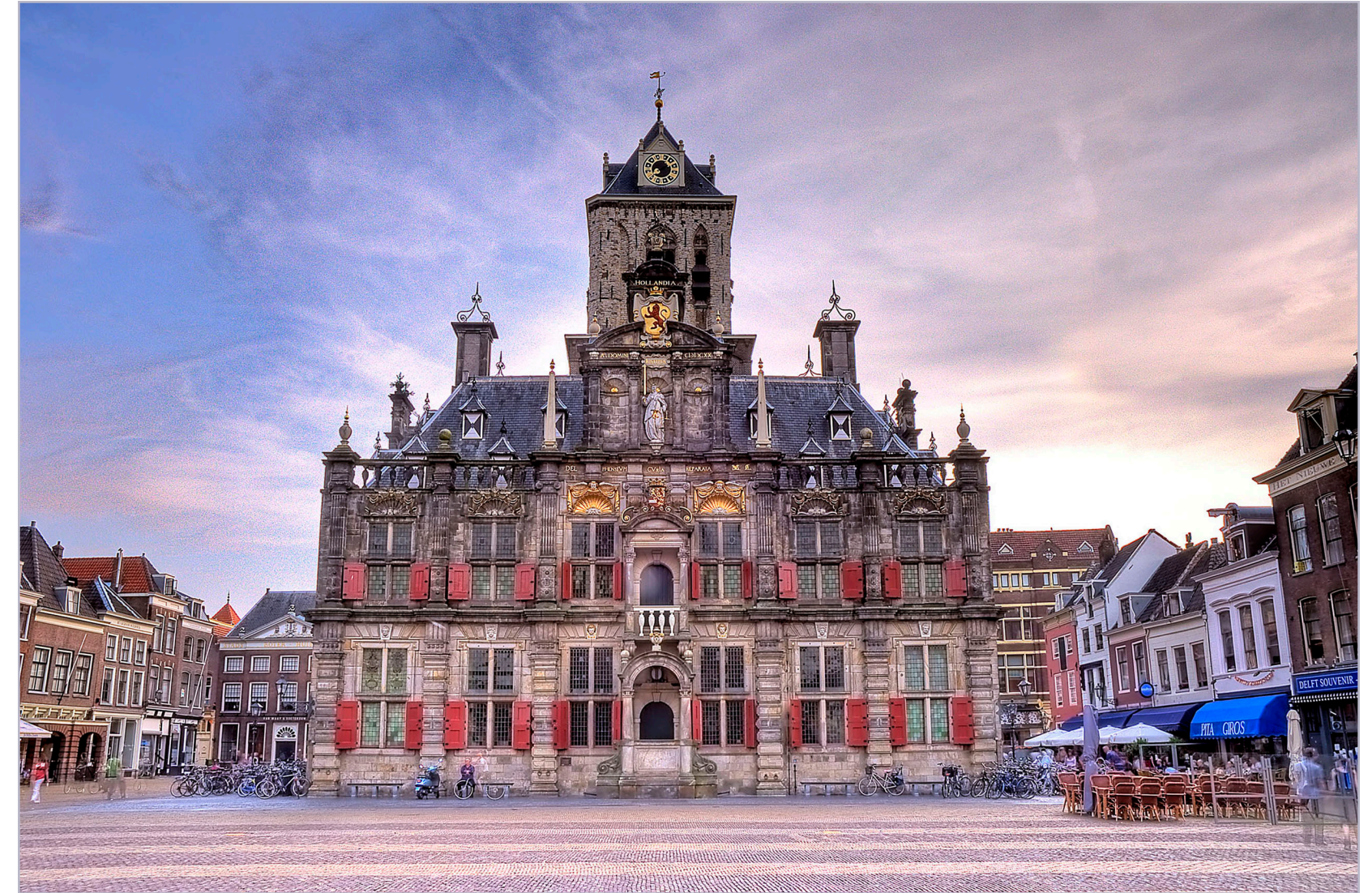
CITY HALL, DELFT, THE NETHERLANDS
